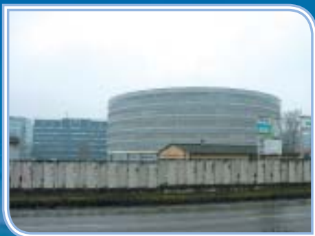
SPP Bratislava Multi-garages
