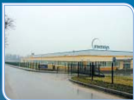
INVENSYS, Trnava Execution of roof damp-proofing
