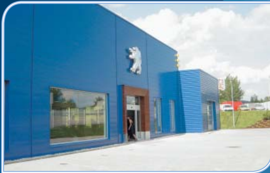
Autocentrum Peugeot Banská Bystrica Execution of fasade and roof insulation
