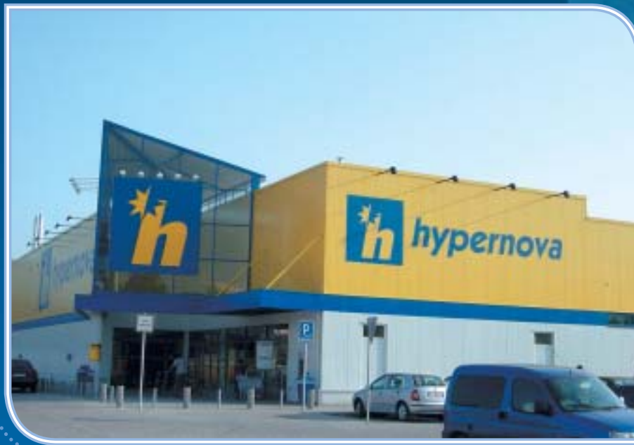
HYPERNOVA Bardejov Execution of roof cladding
