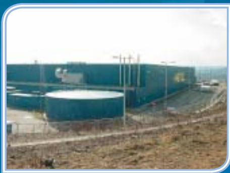
METRO Košice An above-the-ground reservoir, sheathing
