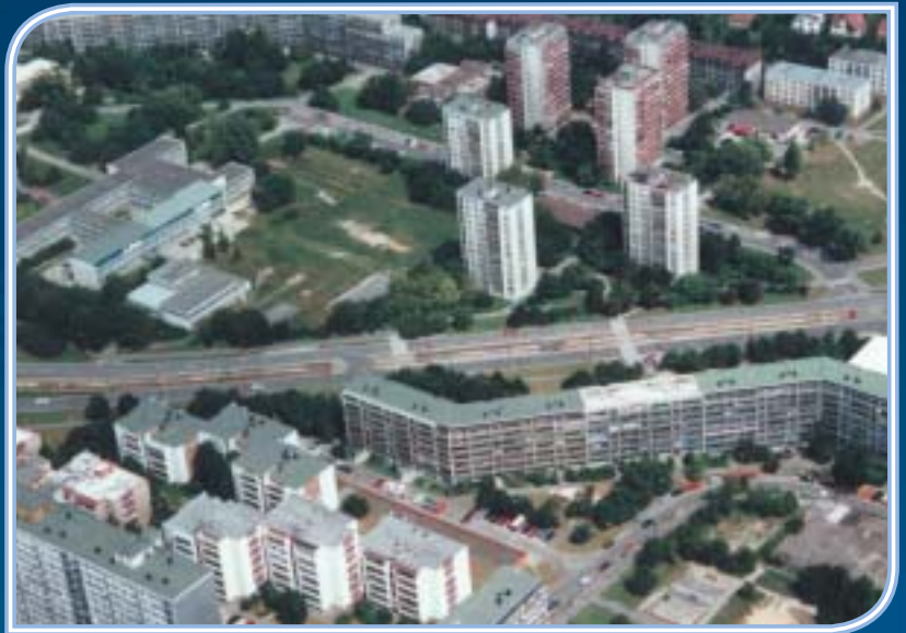
Air photo, Bratislava - Karlova Ves Damp-proofing repairs of roofs
